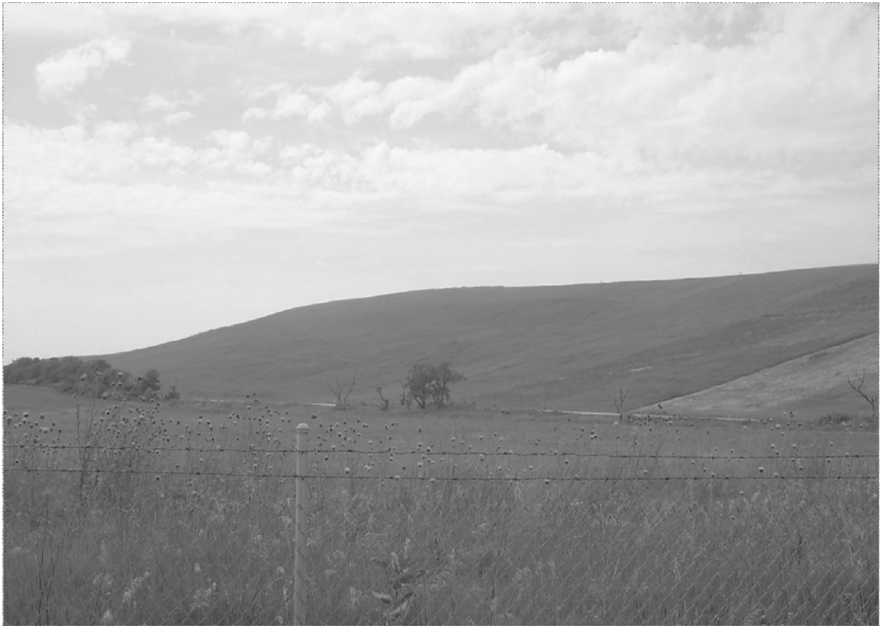
This is not a moraine. While its overall form may resemble a terminal moraine formed by glaciation, this mound lying along the Lisle Township (Du Page County) and Du Page Township (Will County) border is a landfill. It is located at the southern end of the Greene Valley Forest Preserve of the Du Page County Forest Preserve District.
